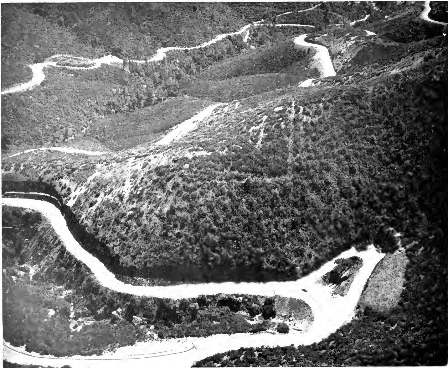
Priests Grade, showing curve correction typical of this project
